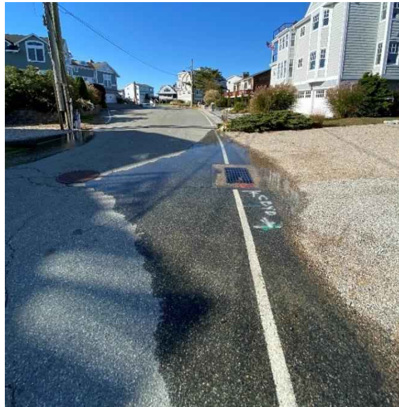
Figure 7: Sunny Day Flooding of Stormwater System (January 2025)
